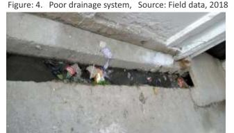
solution can dump lots of excess water into the soil surrounding your home. This excess moisture can cause clay soils to expand, often causing that part of your foundation to "heave" upward or settle. This can result in the same loss of support or stability of your foundation and leave cracks in your interior walls or exterior brick. Mostly drainage lines are filled with garbage and waste materials which often lead to flooding in the rainy season.
